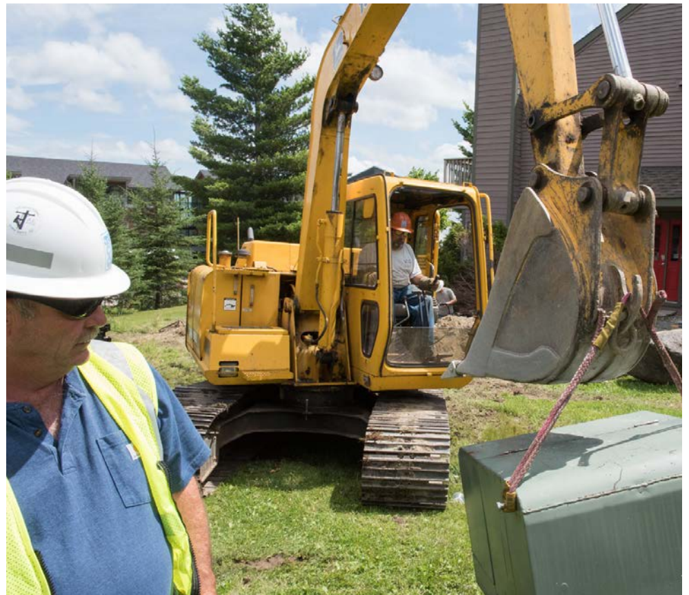
Pad mount transformers, such as this one being moved at Jay Peak Resort, are among the types of equipment that is being affected by supply chain challenges.
